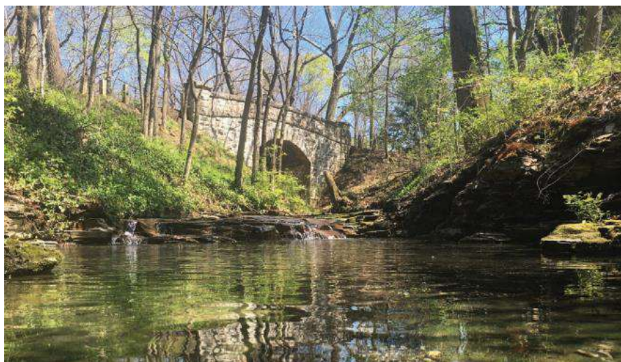
Former zoo bridge situated between the protected areas of Beechwold Nature Preserve.
