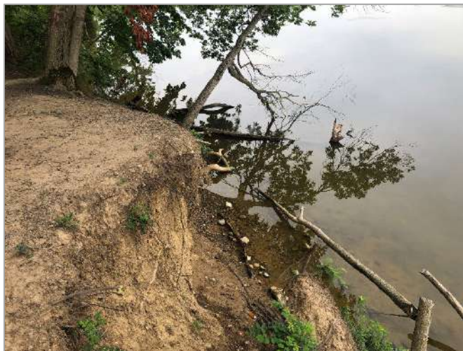
Excessive erosion along Hoover Oxbow's shoreline abutting Hoover Reservoir.
