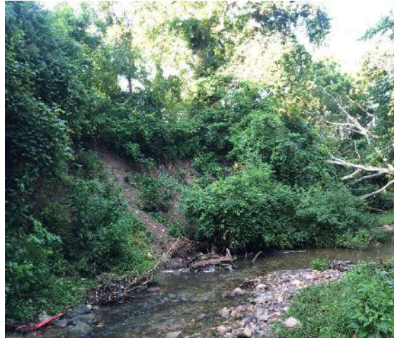
Incised banks and steep erosion along Rush Run.
