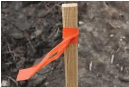
Figure 1- Linear alignment ribbon staking may be helpful during detailed design to help the Natural Resource Professional visualize the alignment in the field.
