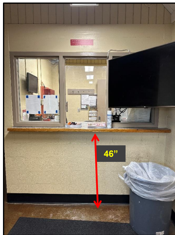
FIGURE 1. COUNTER SPACE GREATER THAN 36 INCHES (BILL MCDONALD ATHLETIC COMPLEX)
