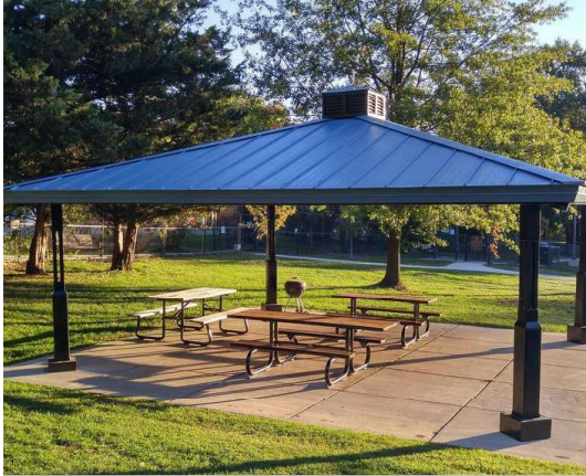
MODERN - STEEL PICNIC SHELTER
