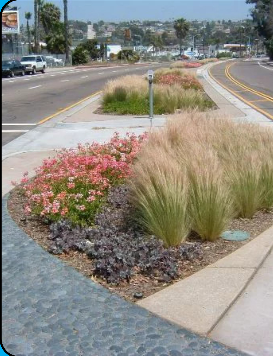
SHRUBS AND TREES NEAR CROSSING
