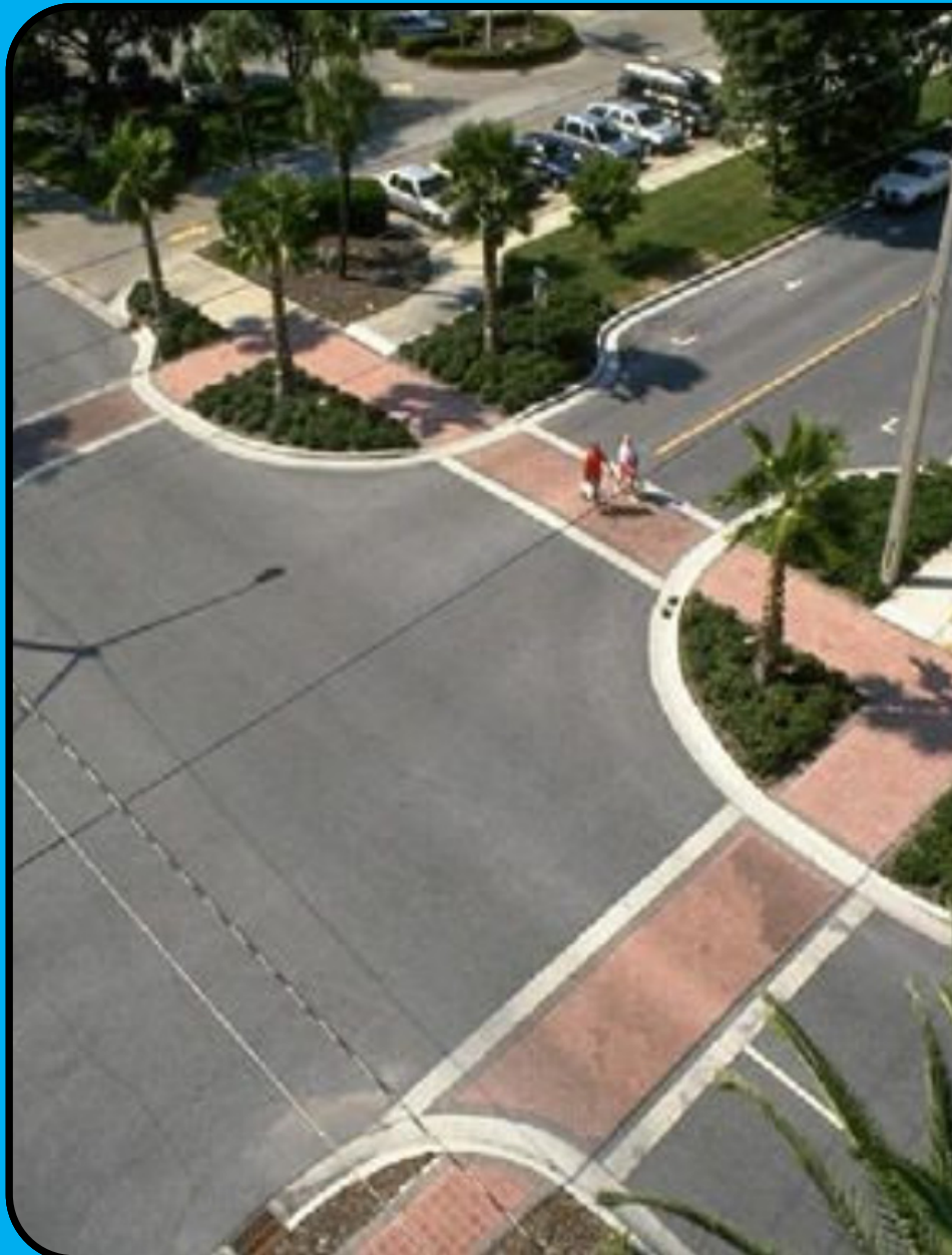
CURB EXTENSIONS TO REDUCE CROSSING LENGTH
